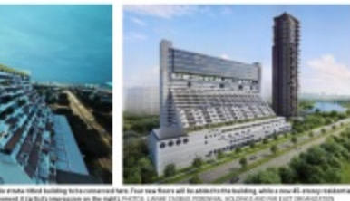
Golden Mile Complex is the first large-scale multi-unit building to be constructed here. Four new floors will be added to the building, while a new 45,000-sq-ft, energy-efficient three-story office building will be built to complement it. It's the first project in the city's history to be built by a private developer, says the city's director of economic development, David L. Smith. The project is being built by the Golden Mile Complex, a joint venture of the city and the private sector.
